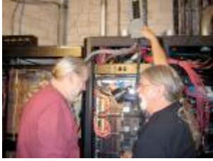
Scott Clarke, technical director, left, inspects the new patch panel and dimmer-per-circuit system with Jackson Lockard, Ventro Electric Company.
